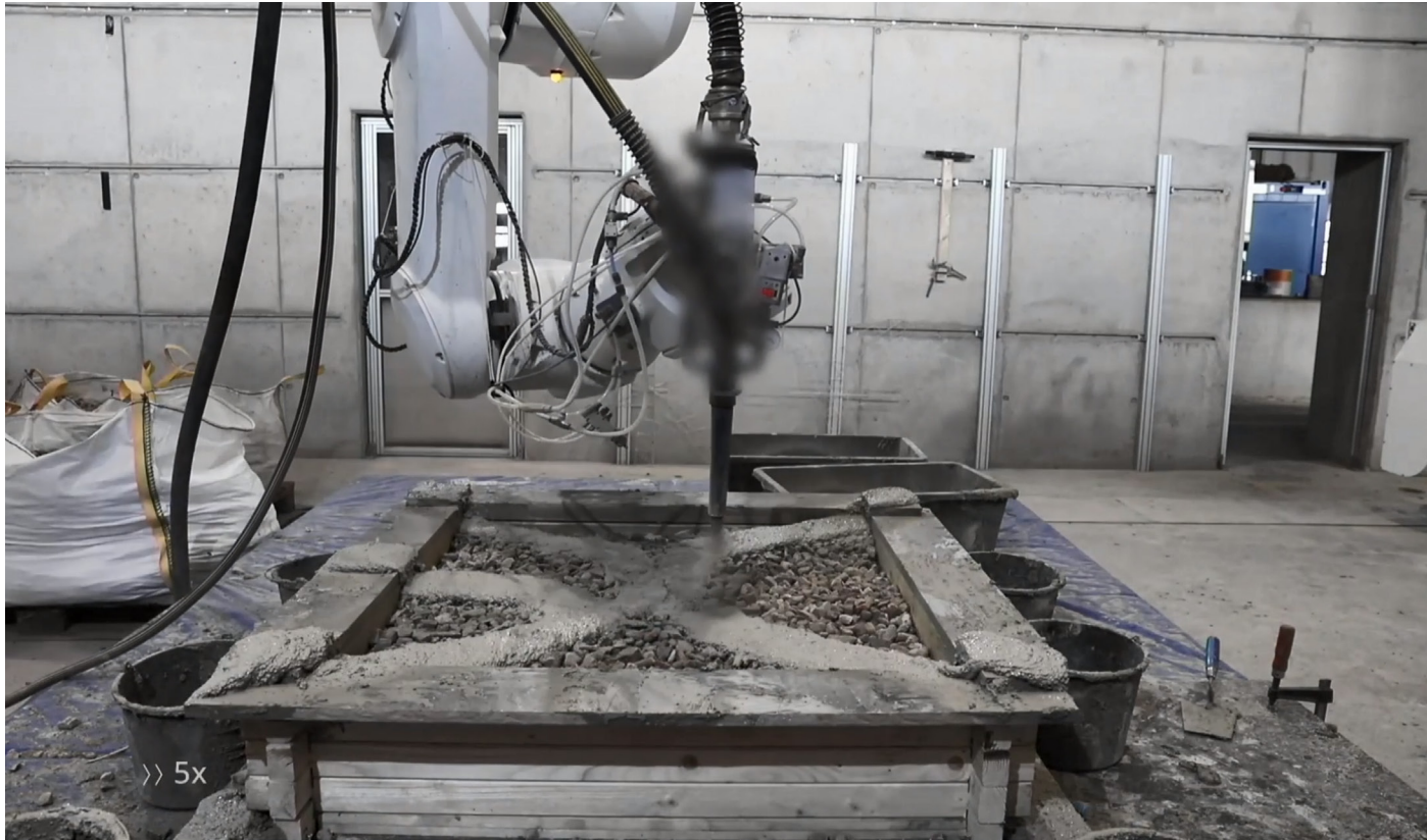
Presentation slide: Prof. Dr. Norman Hack, "The Future of Construction", Zurich 2022: Technische Universität Braunschweig, Robot printing concrete on top of debris, 2022
