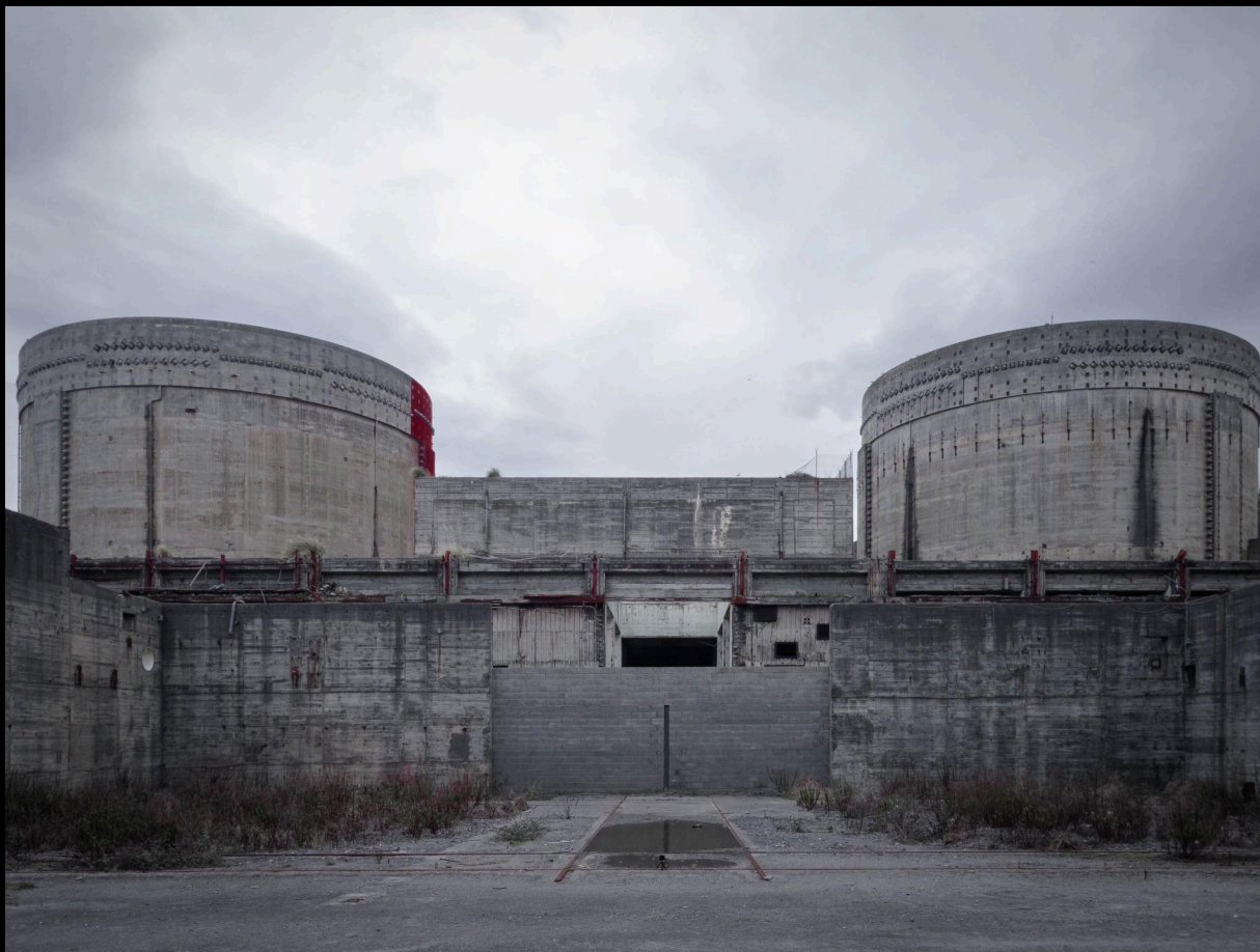
FIG. 2. UNFINISHED NUCLEAR POWER PLANT LEMONIZ, SPAIN
