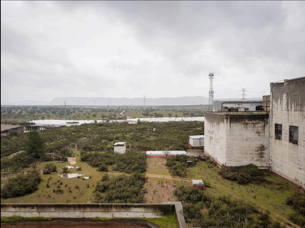
FIG.1. UNFINISHED NUCLEAR POWER PLANT VALDECABALLEROS, SPAIN
